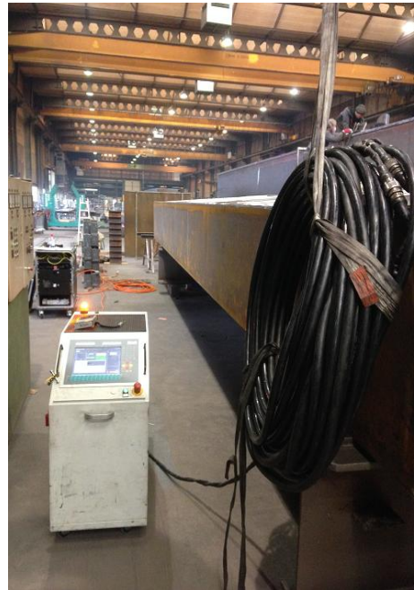
Demagnetization of a steel box girder
